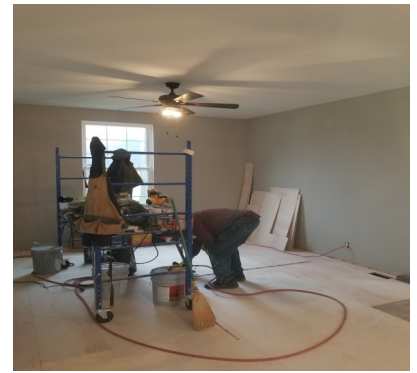
Living room-preparation for new floor
