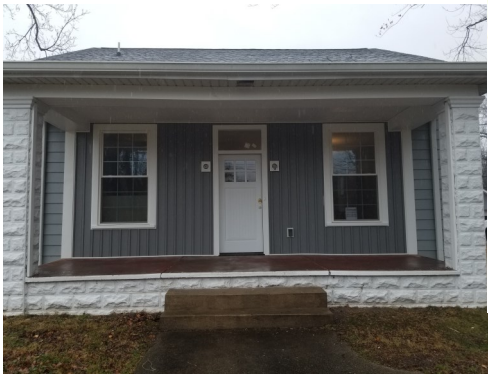
New front/porch of the house
